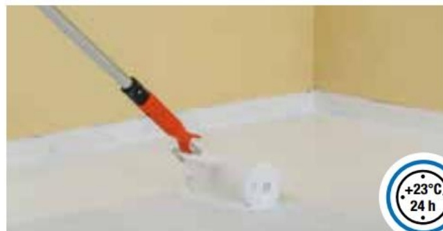
Application of the second coat
