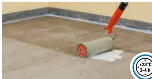
Priming the substrate
