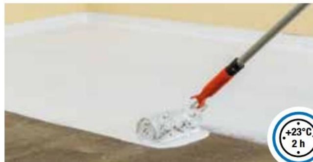
Application of the first coat
